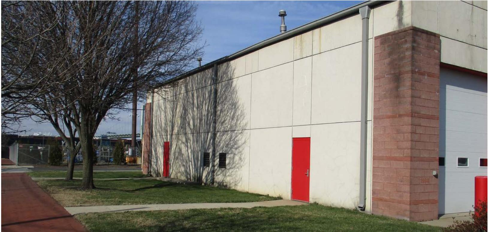
This site is located at the Gloucester City Fire Department. Stormwater is currently draining to nearby catch basins. Downspouts along the building can be directed into rain gardens to capture, treat, and infiltrate runoff. A cistern connected to building downspouts can capture water, allowing it to be used for washing vehicles and equipment.
