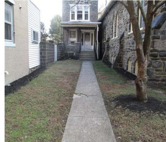
Stormwater is currently draining from north to south across the site. A stormwater planter can be constructed along the southern sidewalk to capture and treat stormwater runoff. Downspouts along the building can be directed into rain gardens. Installing rain gardens adjacent to the building can capture, treat, and infiltrate runoff. A preliminary soil assessment suggests that more soil testing would be required before determining the soil's suitability for green infrastructure.
