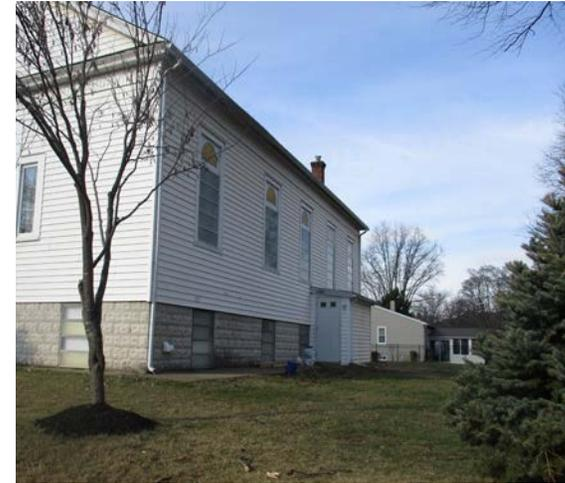
Stormwater is currently draining from east to west across the site. Building downspouts can be directed into a rain garden. Installing a rain garden adjacent to the building can capture, treat, and infiltrate roof runoff. A preliminary soil assessment suggests that more soil testing would be required before determining the soil's suitability for green infrastructure.
