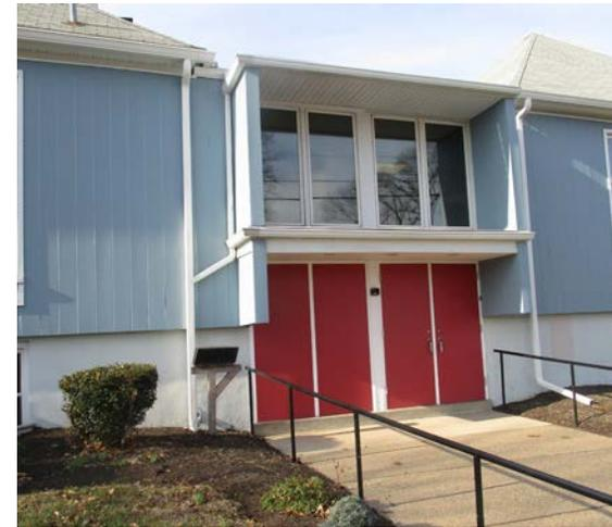
Stormwater is currently draining across the site to nearby catch basins. Building downspouts can be disconnected and directed into a rain garden. Installing a rain garden adjacent to the building can capture, treat, and infiltrate roof runoff. A preliminary soil assessment suggests that more soil testing would be required before determining the soil's suitability for green infrastructure.
