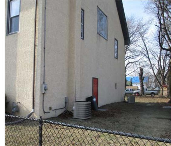
Stormwater is currently draining across the site to nearby catch basins. Building downspouts can be directed into a rain garden. Installing a rain garden adjacent to the building can capture, treat, and infiltrate roof runoff. A preliminary soil assessment suggests that more soil testing would be required before determining the soil's suitability for green infrastructure.
