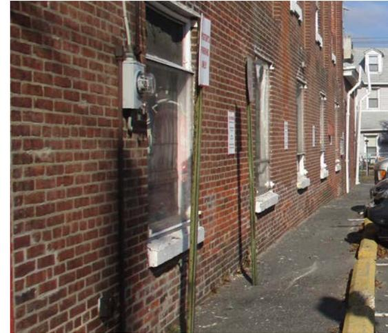
Stormwater is currently draining from south to north across the site. Parking spaces in the east lot can be converted to porous asphalt to capture and treat stormwater runoff. Adjacent downspouts along the building can also be directed into the parking lot, allowing for the treatment of roof runoff. A preliminary soil assessment suggests that more soil testing would be required before determining the soil's suitability for green infrastructure.
