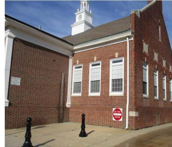
Stormwater is currently draining from south to north across the site. Paved areas to the east and west and of the south entrance can be converted to porous asphalt to capture and treat roof runoff. A preliminary soil assessment suggests that more soil testing would be required before determining the soil's suitability for green infrastructure.
