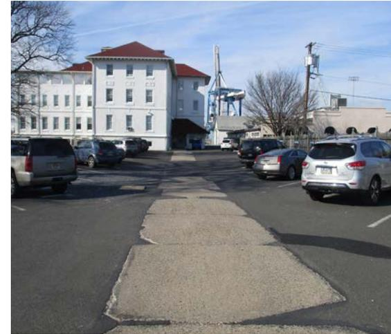
Stormwater is currently draining across the site into nearby catch basins. Parking spaces in the east lot can be converted to porous asphalt to capture and treat stormwater runoff. Stormwater can be diverted from the main parking lot into a rain garden. Installing a rain garden adjacent to the parking lot can capture, treat, and infiltrate runoff. A preliminary soil assessment suggests that more soil testing would be required before determining the soil's suitability for green infrastructure.
